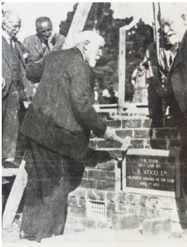
1927 L.B. Wood, laying the foundation stone for the new clubhouse
